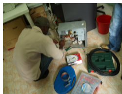
Wireless adaptor installation at Chóckwe
