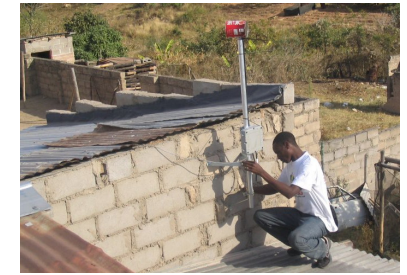
Community member installing a WiFi node with antenna
